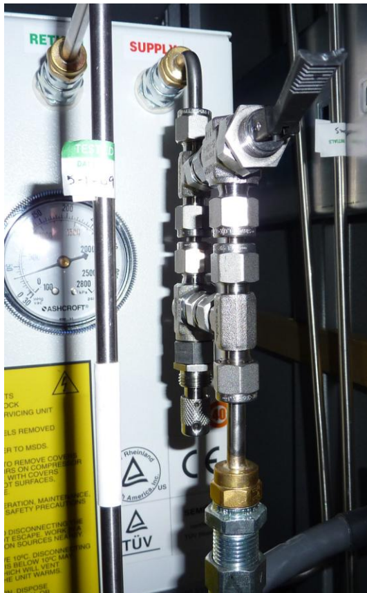
Figure 38 - Flow unrestricted position (for cooldown)
