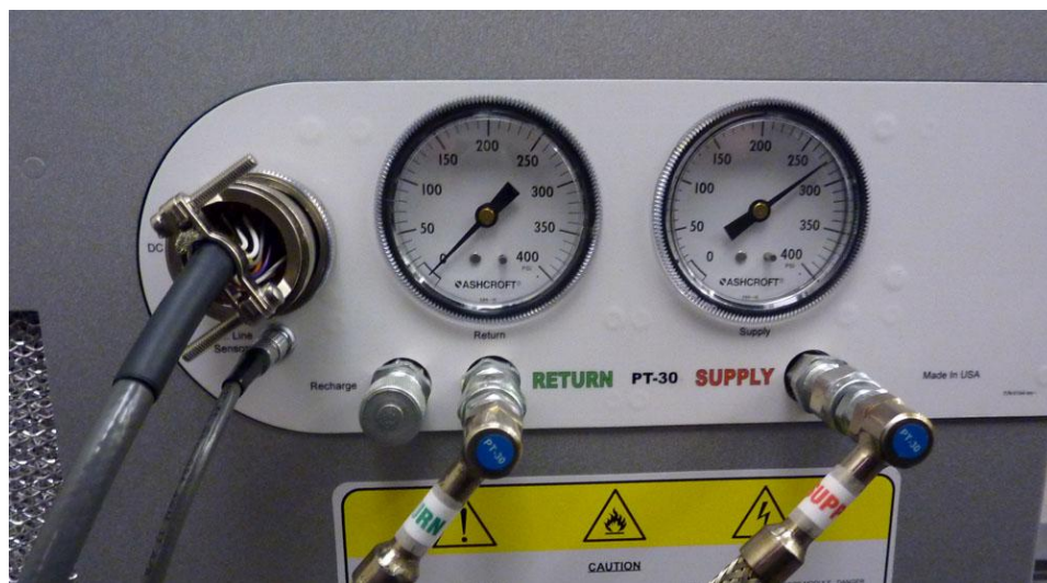
Figure 36 - SX Series cabinet connections
